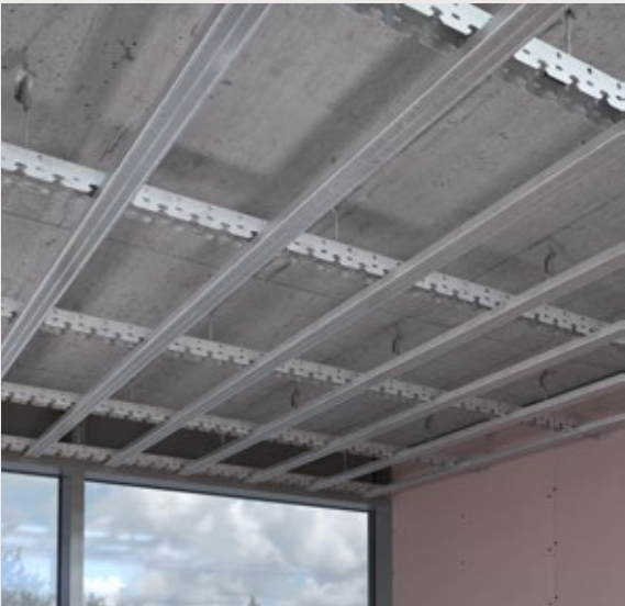
The primary metal frame is laid with a 50-60 cm pitch and the secondary with a 30 cm pitch. This step ensures that the panel is properly anchored, and, in the wall application, also makes it shatterproof.
