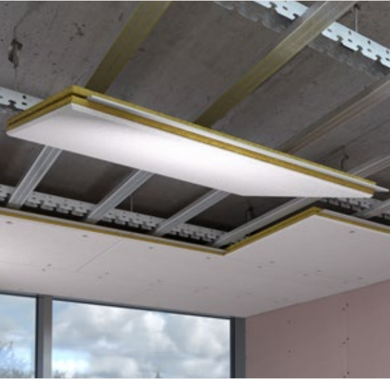
1A. The panels are then applied to the metal frame, securing them with self-tapping screws and washers. A perimeter ridge (male-female system) facilitates the support of the next panel when fixing panels with screws.
