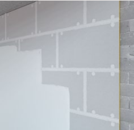
2. Grout joints and screw holes with INN Putty then when completely dry, apply a first coat of INN Fin skim coat.
