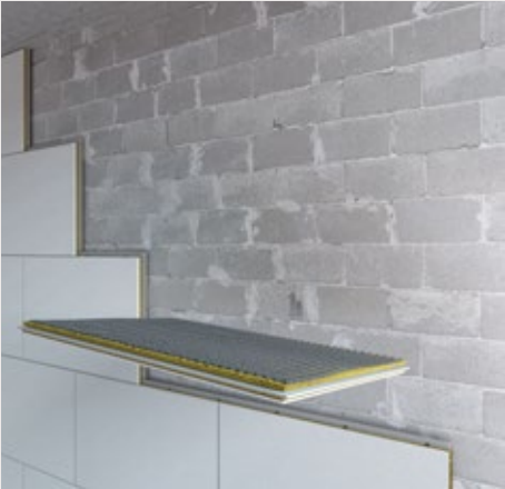
1. INN Colfiss cement glue application and fixing panels with suitable dowels and plugs.
