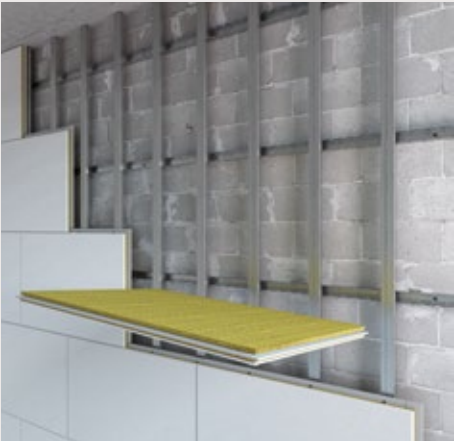
1. Fastening panels to the frame with screws on the ridge.
