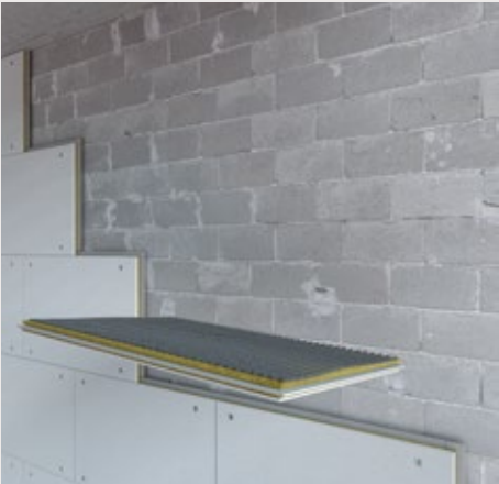
1. Application with INN Colfiss cement glue and panel fixing with dowels and washers.
