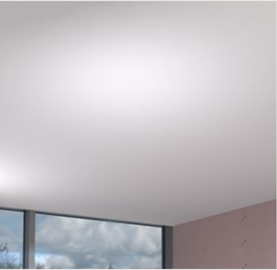
3. Finally, once the first skim coat is perfectly dry, you can proceed with the final coat, again using INN Fin . The finish is supplied coloured in a paste.
