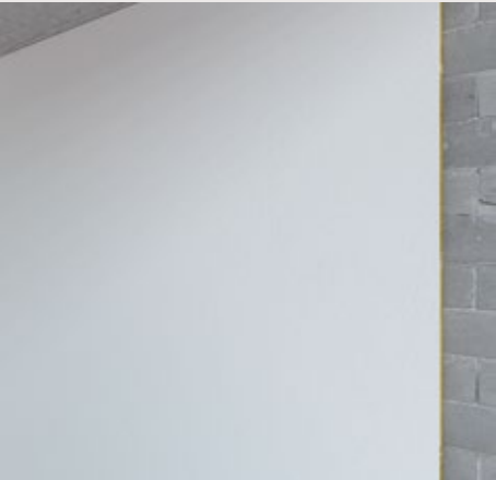
3. When completely dry, apply second coat of INN Fin skim coat.
