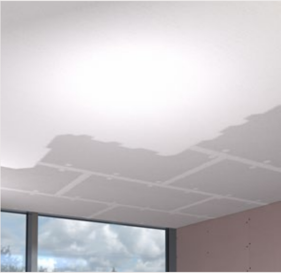
2. When the grout is perfectly dry, you can proceed with a first skim coat using our specially formulated product, INN Fin .
